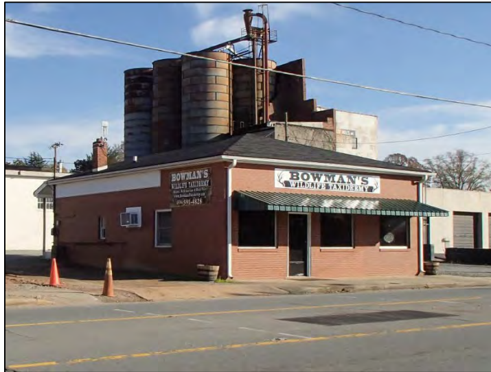
Figure 12: 416 North Main Street
