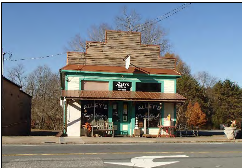
Figure 29: 409 North Main Street
