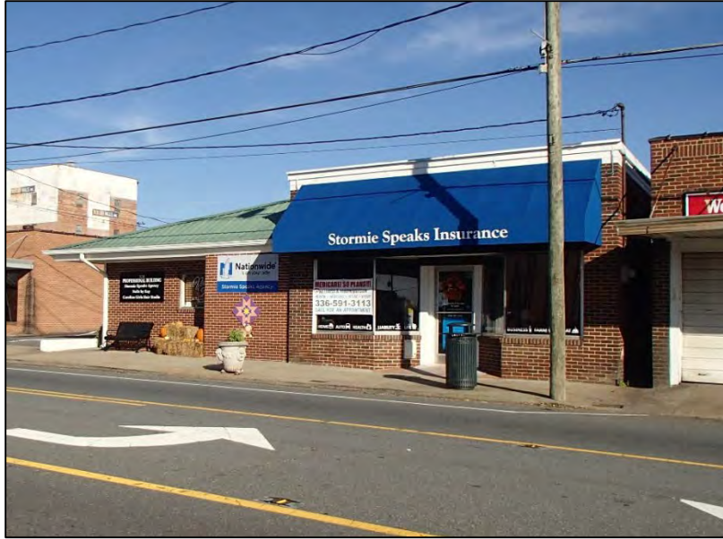
Figure 8: 328-330 North Main Street
