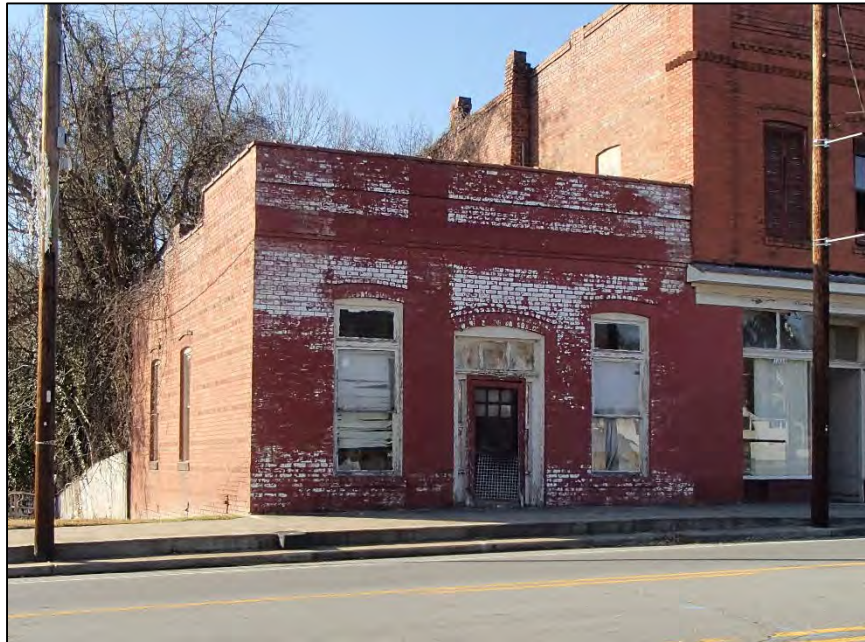
Figure 14: 133 North Main Street
