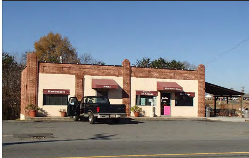
Figure 30: 419 North Main Street
