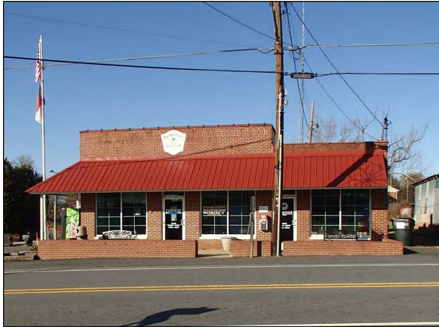
Figure 32: 208 West Third Street
