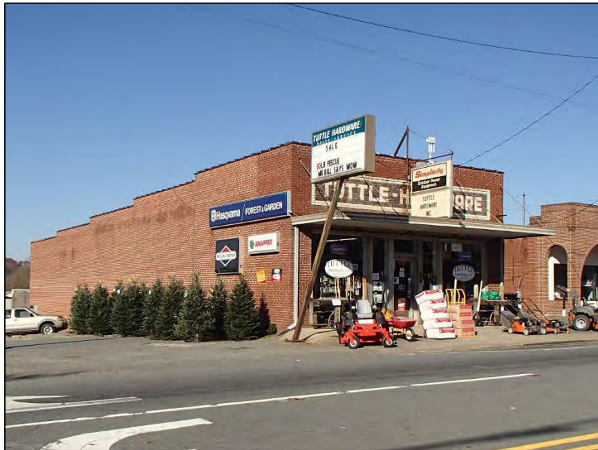
Figure 22: 311 North Main Street
