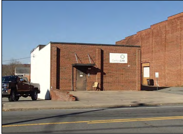
Figure 24: 323 North Main Street
