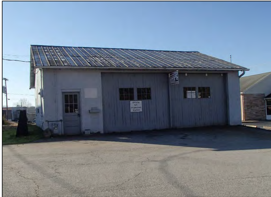
Figure 35: 104 West Fourth Street
