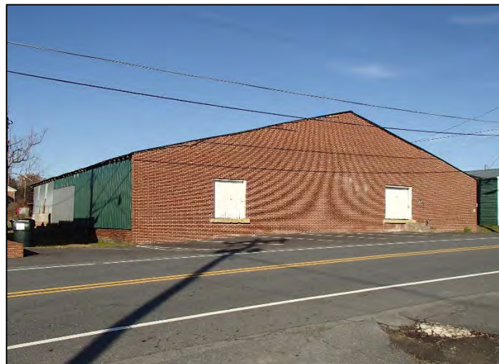
Figure 31: 204 West Third Street
