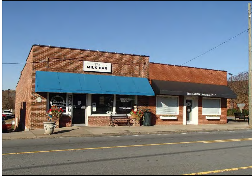
Figure 18: 213 (left) and 215 (right) North Main Street
